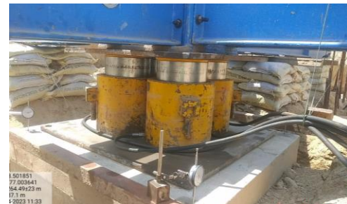
(b) Close-up view showing hydraulic jacks and dial gauges
