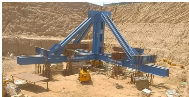
(a) Truss with 16 anchor piles installed over the footing
